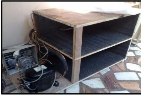
Fig. 1 Practical Implementation of the cooling system.
